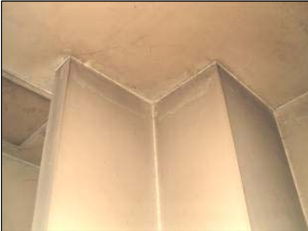
A photo of the impact of the kerosene stove on the wall.
